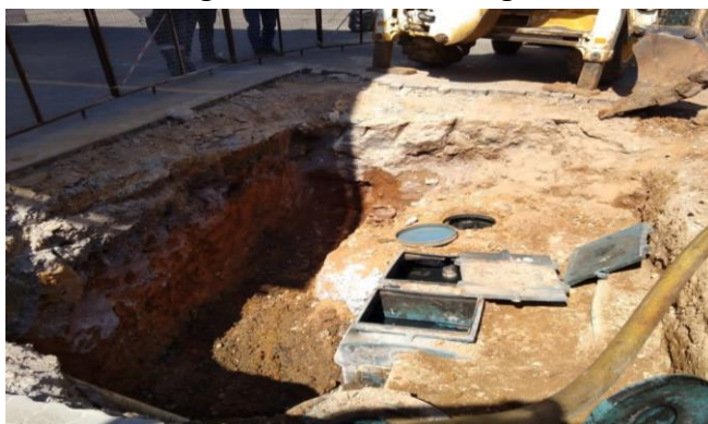
2020 – Underground Tanks cleaning & removal
